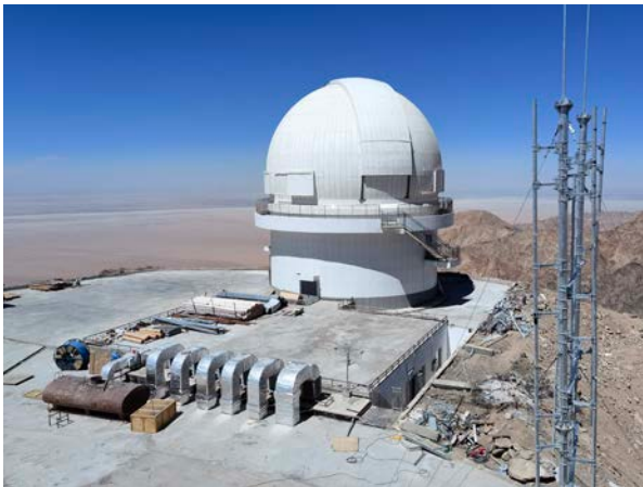
This photo, taken on 16 August 2023, shows the Wide Field Survey Telescope (WFST) in Lenghu Town in northwest China's Qinghai Province. A wide-field telescope measuring 2.5 meters in diameter, WFST is capable of surveying the entire sky from the Northern Hemisphere. | Image Source: AFP; Xinhua
